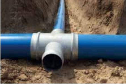
CONDUTAS EM TUBO PVC Dn315-250-200 E 160MM Pn6 COM EXTENSÃO TOTAL DE 2694 METROS
